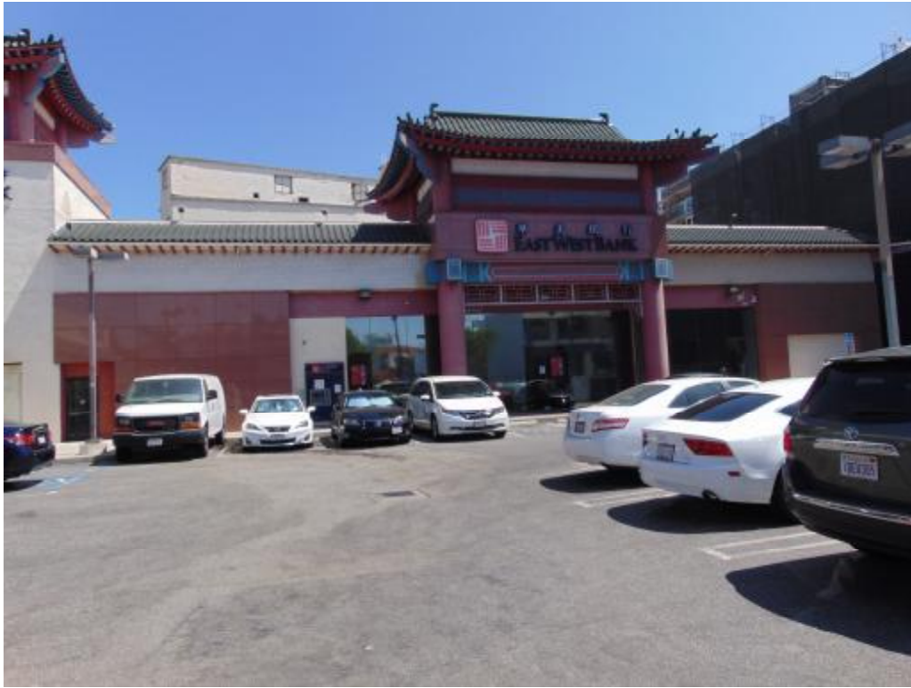
Photograph No. 1: View across the front parking lot toward the bank.
