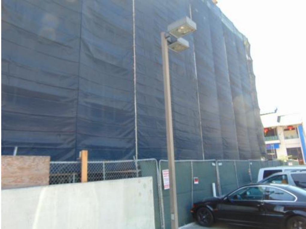
Photograph No. 13: The southwest-adjacent construction site as seen from the property.
