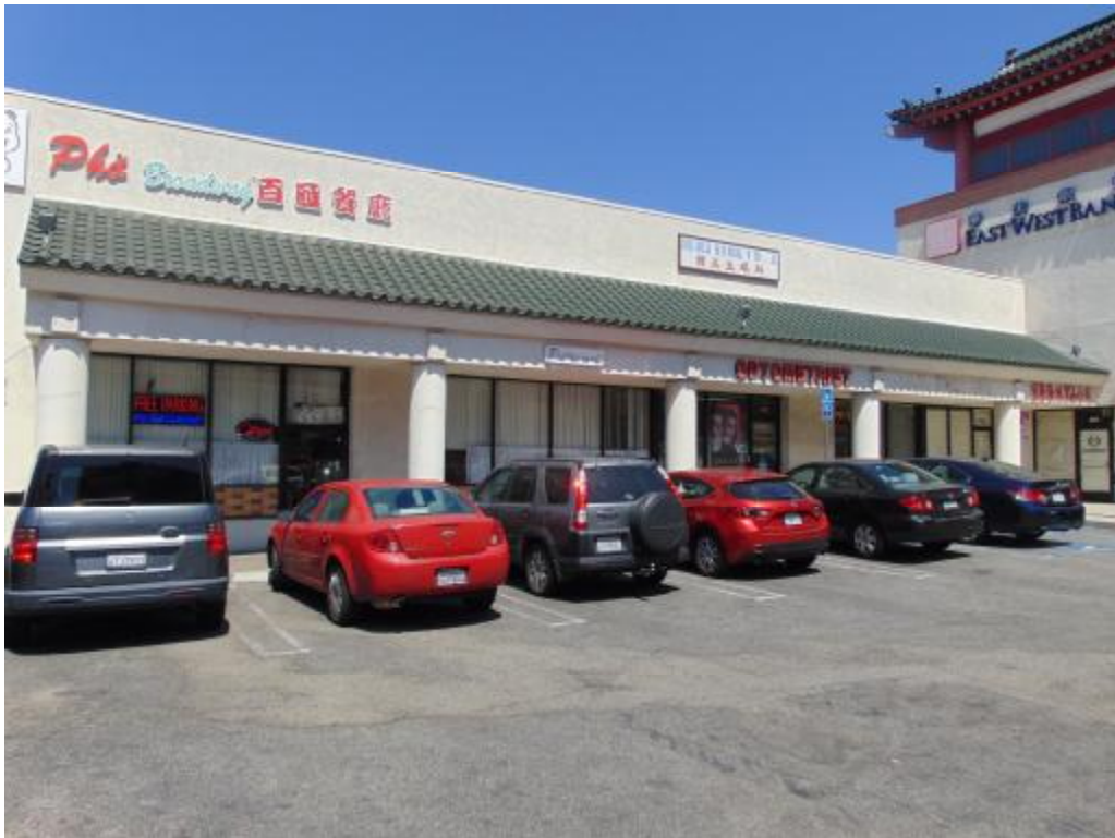
Photograph No. 2: View of the multi-tenant retail portion of the property.
