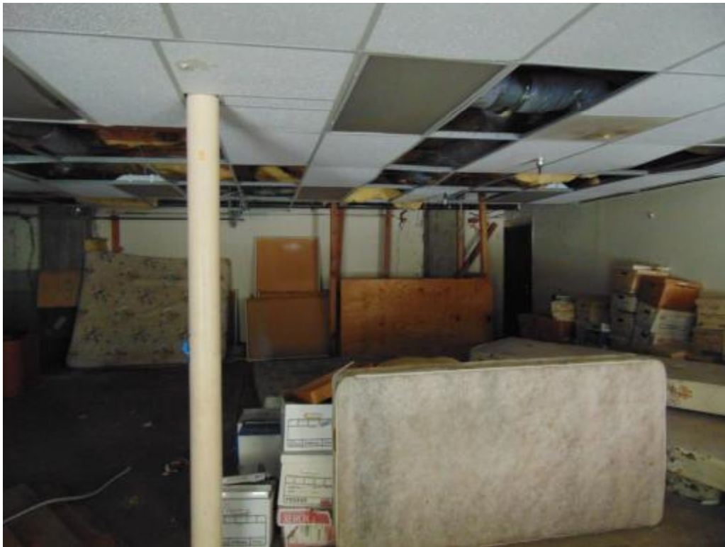
Photograph No. 10: Another storage area in the basement.
